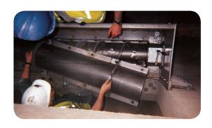
The internal components of the Heliscreen are mounted on the 'wet' (sewer) side of the weir. The main components are easily accessible from the 'dry' side for maintenance or inspection.
